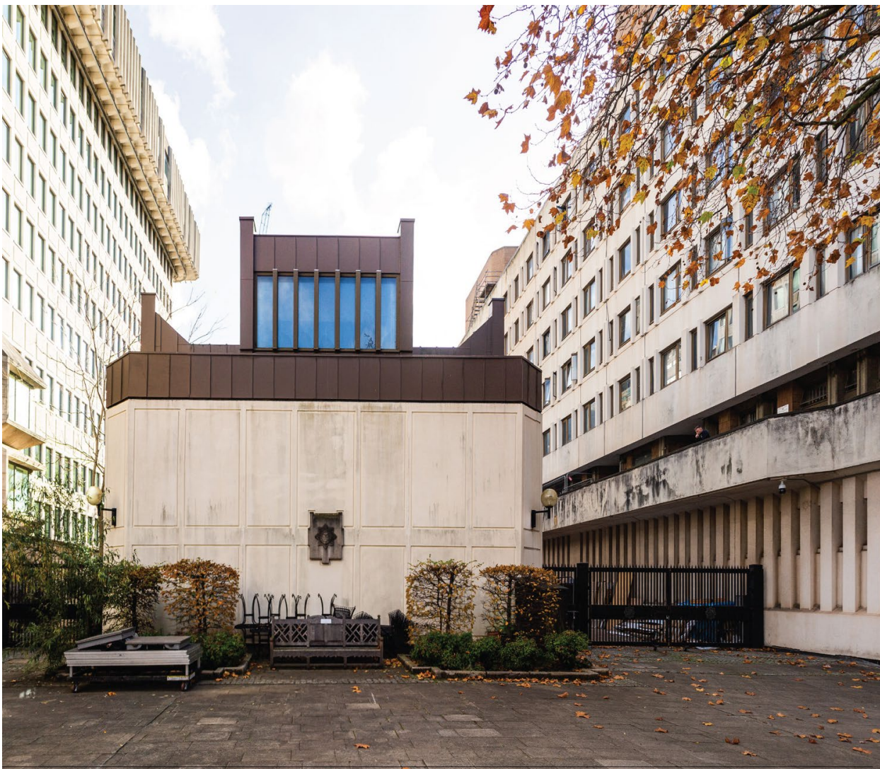
Wellington Barracks Rehearsal Hall, North elevation
