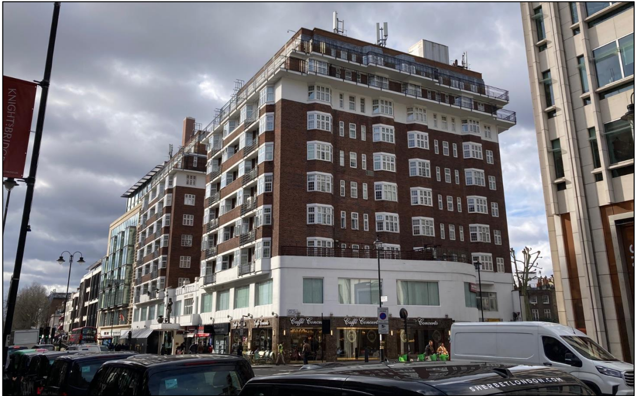
The application site (Princes Court) as seen from the corner of Hans Crescent and Brompton Road
